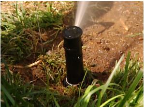
Pop up rotor, note cover plate is flush with grade below turf blades. Picture by diynetwork.com
