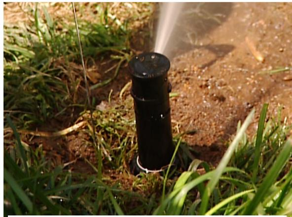
Pop up rotor, note cover plate is flush with grade below turf blades. Picture by [diynetwork.com](http://diynetwork.com)
