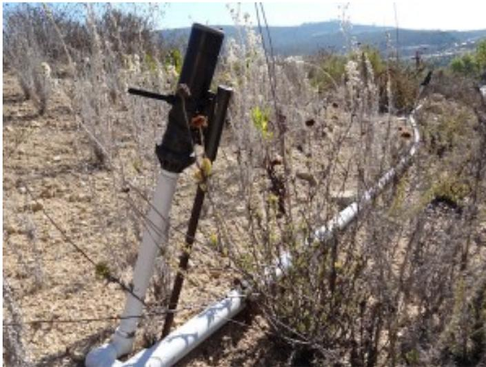
**A staked rotor head on riser should be used where no pedestrian traffic occurs.**
