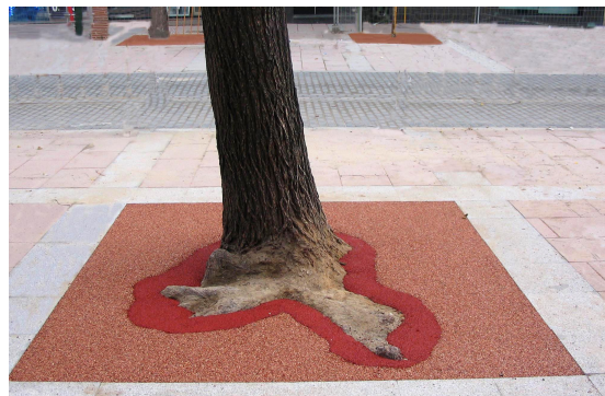
Safe Path installed around tree collar and surface roots. Photo by Blue Drop
