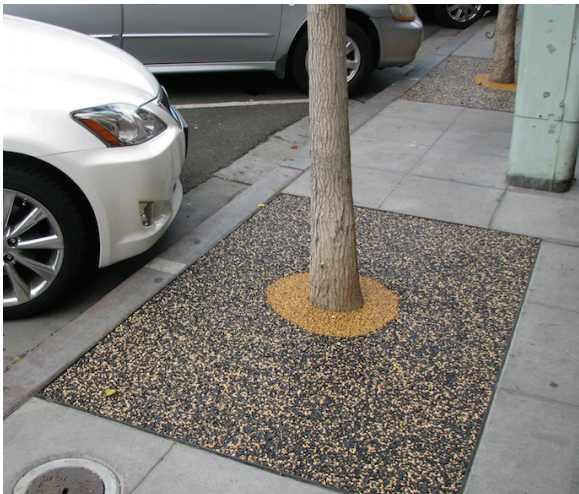
A tree planter with Safe Path product replaces cast iron tree grate. Photo provide by Blue Drop, Inc.
