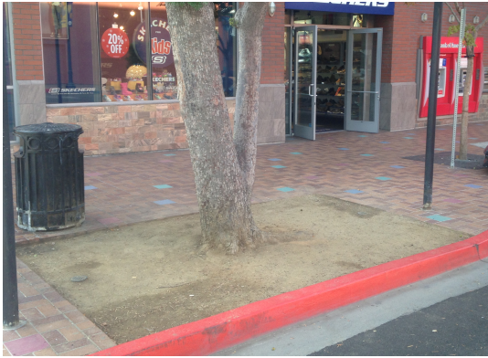
Old grate and sidewalk removed, planter is prepped for Safe Path. Photo by Blue Drop
