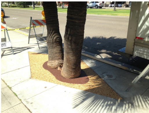
Safe Path installed in diamond planter configuration. Photo by Blue Drop
