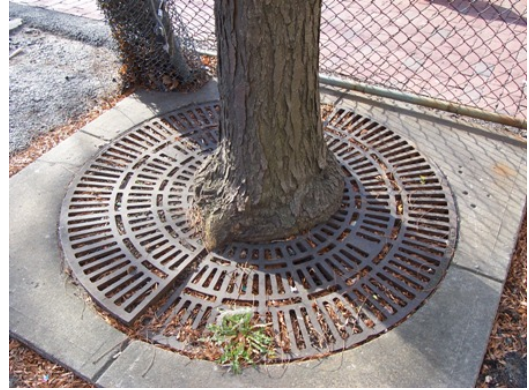
Tree lifts one side of a grate creating a trip and fall hazard. Photo by localecologist.blogspot.com
